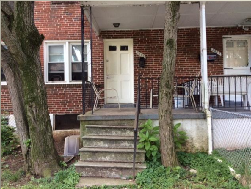
MOG house on Oswego with gas leak
